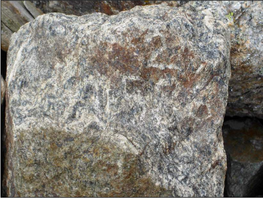
Close-up photograph of the west, sloping face that is chiseled "2 - 15889."
