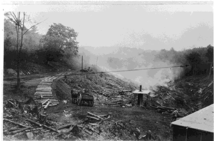
Construction of the Dam in 1923, courtesy of NHDES Files
