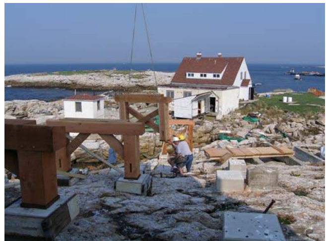
Setting the timber trestles.
